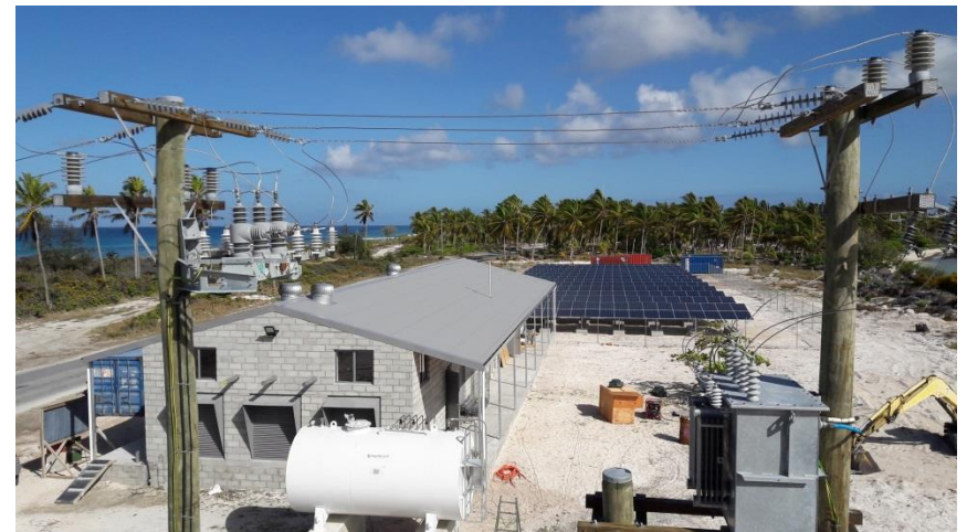
Figure 1.4 Through our subsidiary Infratec we are involved in new technology projects such as this solar power station in Kiritimati.
