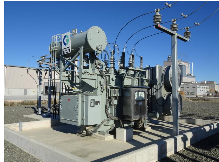
Figure 6.18 Zone substation transformer – Cooneys Road substation
