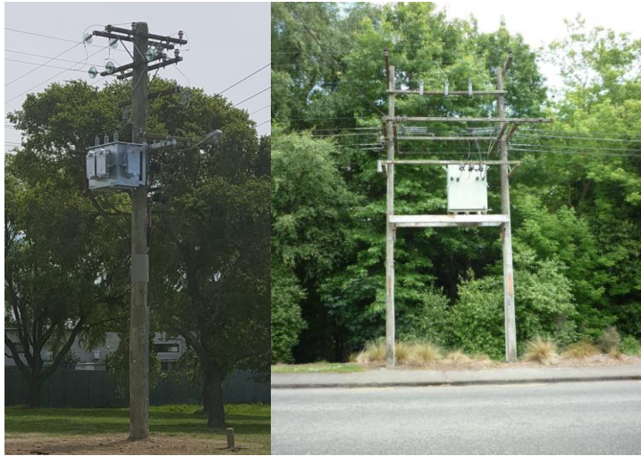
Figure 6.32 Pole mounted distribution transformers
