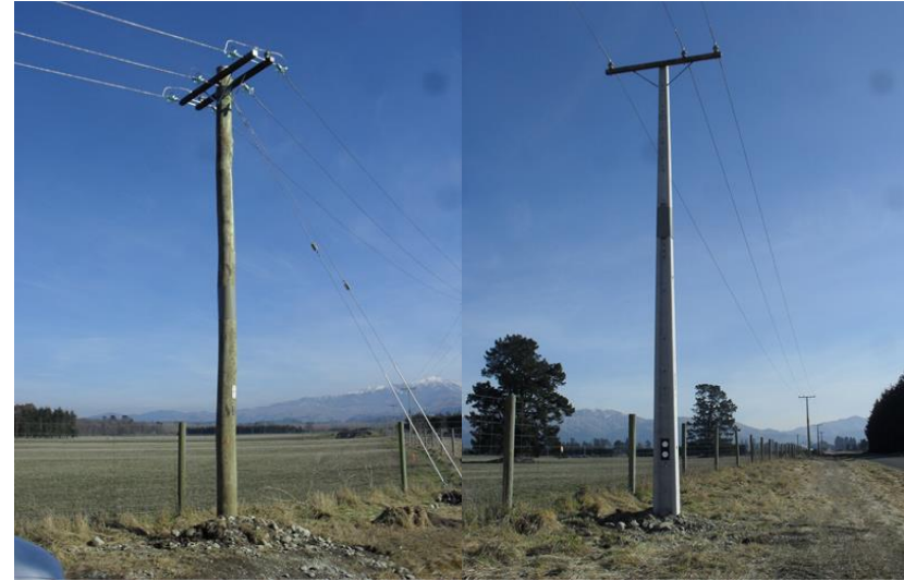
Figure 6.6 Wood pole left and concrete pole right.
