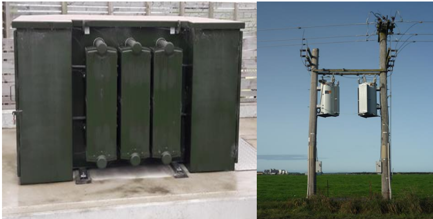
Figure 6.32 Pole mounted distribution transformers
