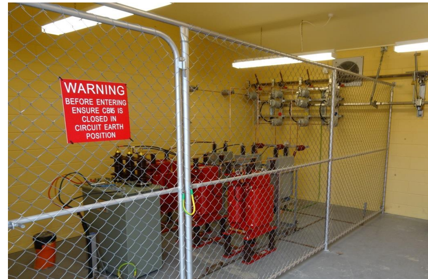
Figure 6.29 Load control injection plant – Bells Pond zone substation
