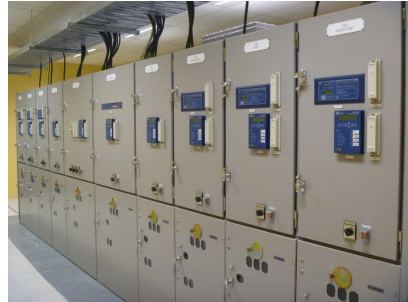
Figure 6.21 11 kV Indoor switchboard at North Street substation
