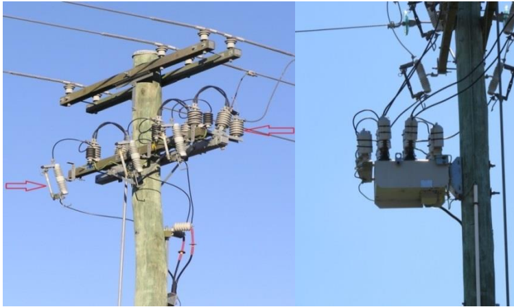
Figure 6.39 Fuse link left and an ABS right
