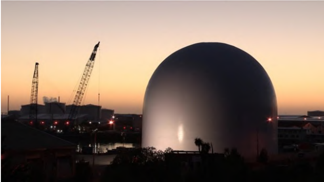
Figure 3.2 Holcim's cement silo
