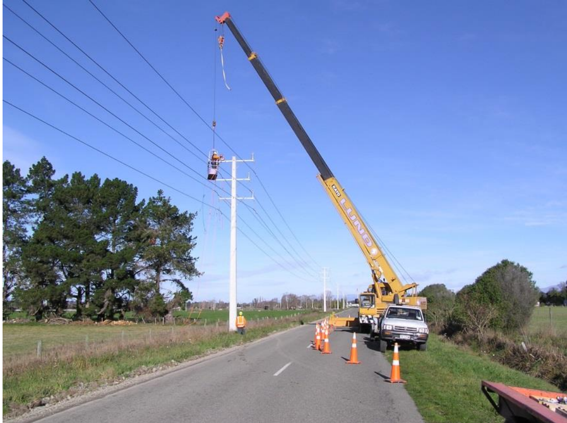
Photograph 3.7 Construction of 33 kV lines to Clandeboye Dairy Factory
