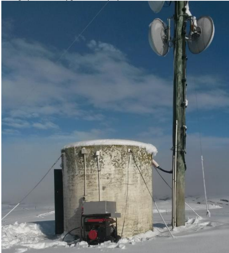
Photograph 3: Standby generator deployed to telecommunications tower
