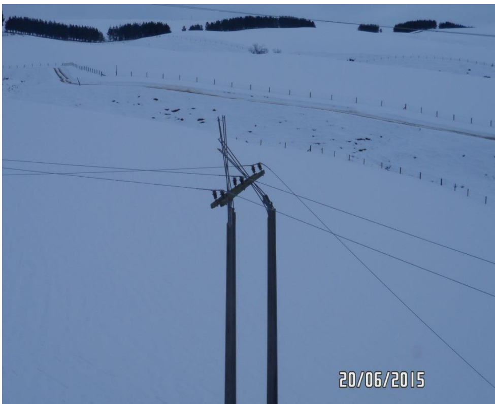
Photograph 6: Example of assets damaged by sticky snow on the lines
