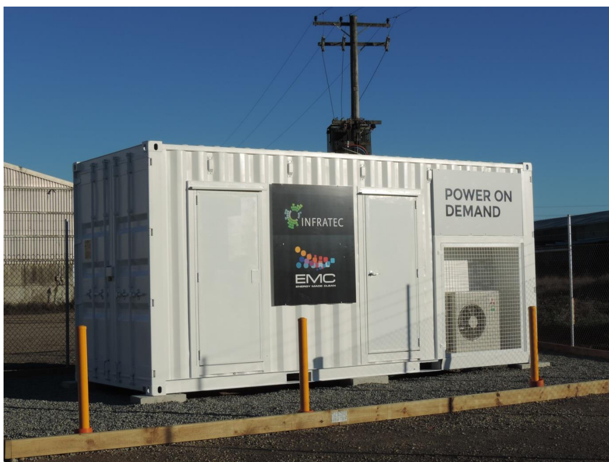
Photograph 13: Containerised battery system
