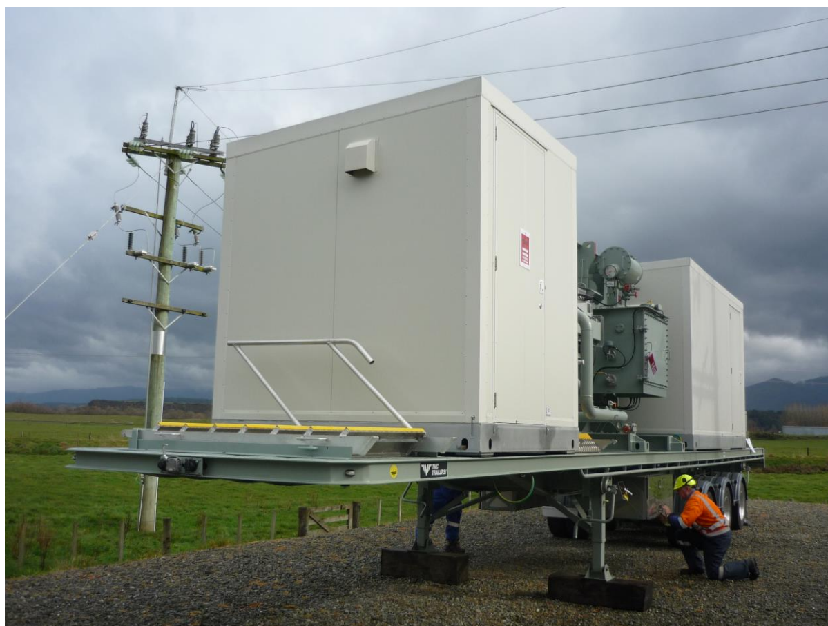
Photograph 12: Our mobile substation
