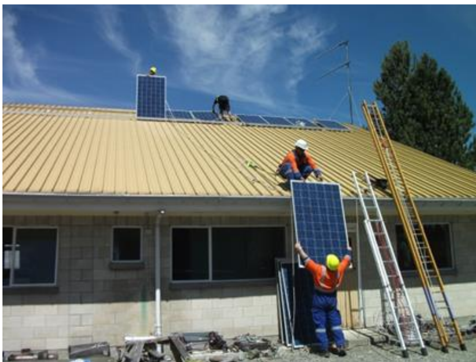
Figure 5.6 Installation of PV panels
