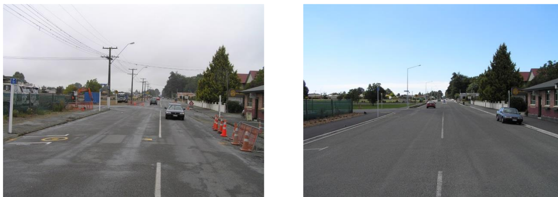
Figure 3.11 Undergrounding LV infrastructure at Domain Road
