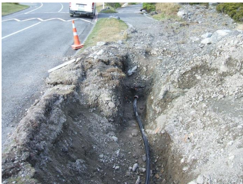
Figure 3.16 Mt Cook Village cable repairs
