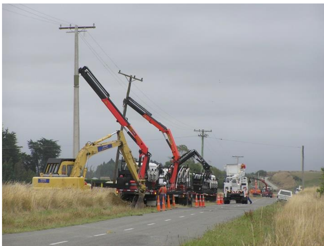
Figure 6.4 Replacing poles
