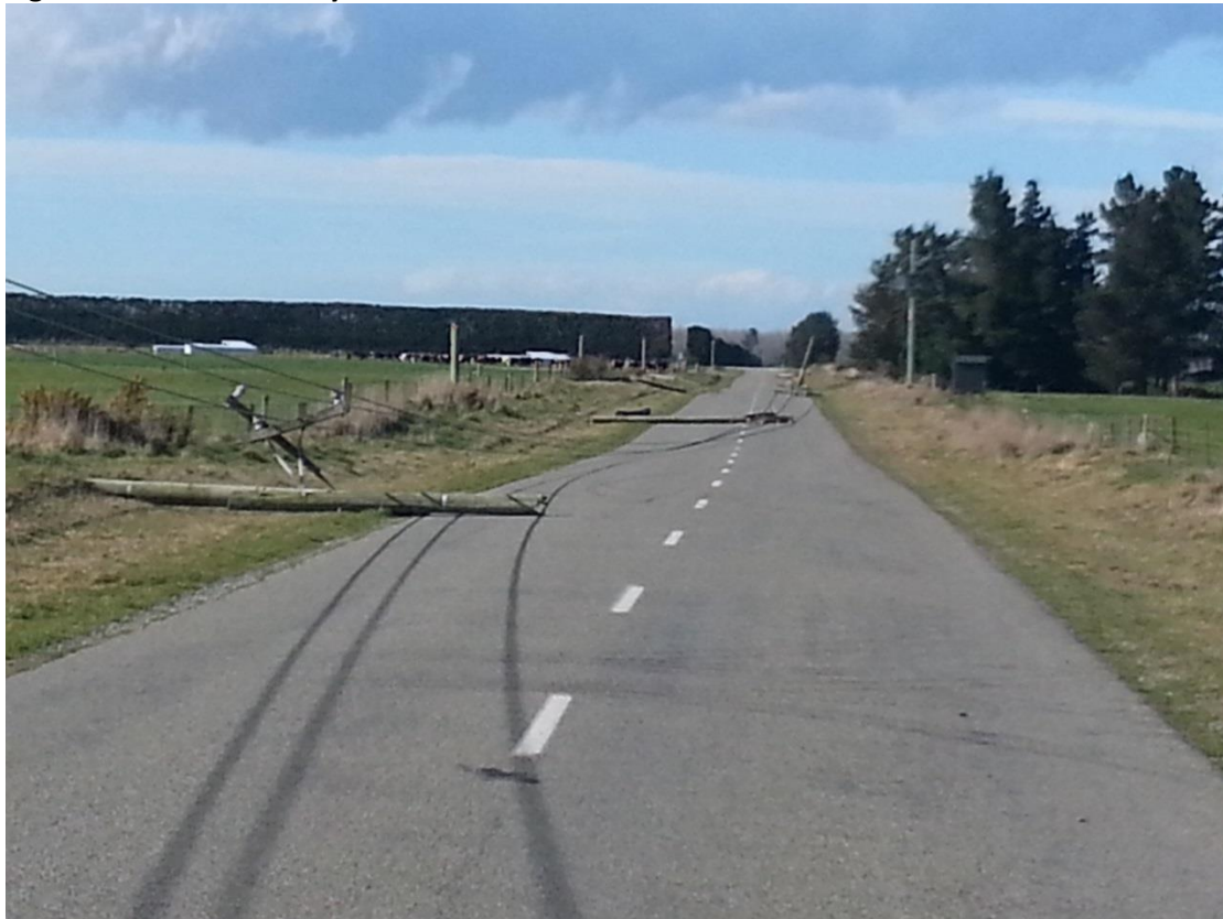
Figure 7: Poles broken by wind storms
