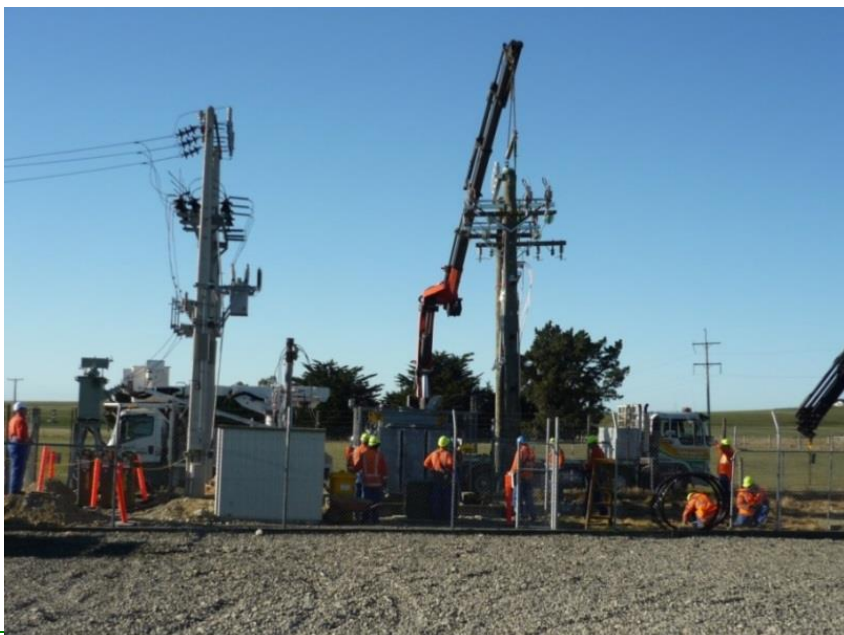
Photograph 2.1 Albury Step-up Structure 2012 Upgrade in Progress
