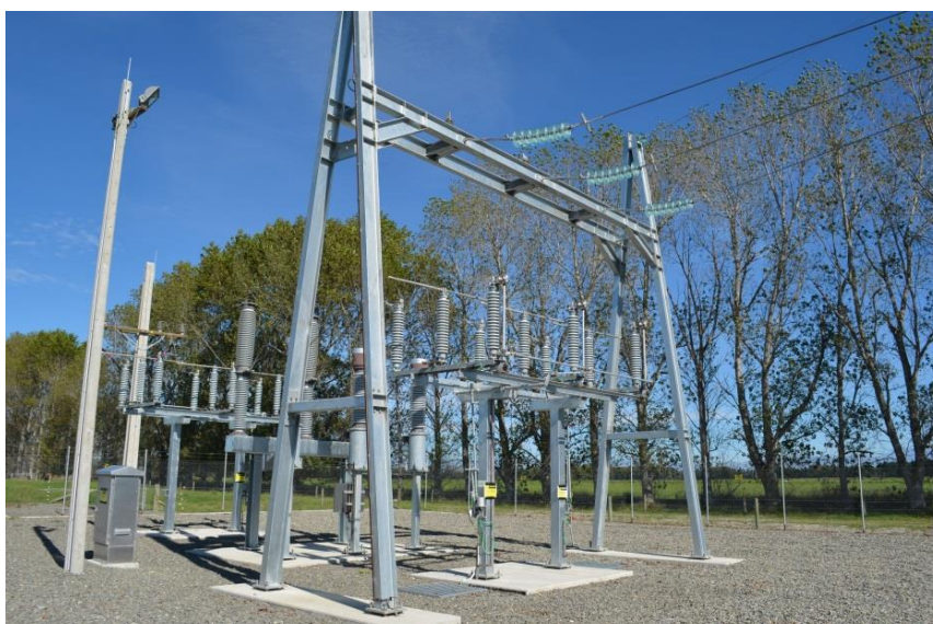
Photograph 3.3 Bell's Pond 33 kV Terminal for CNRs line
