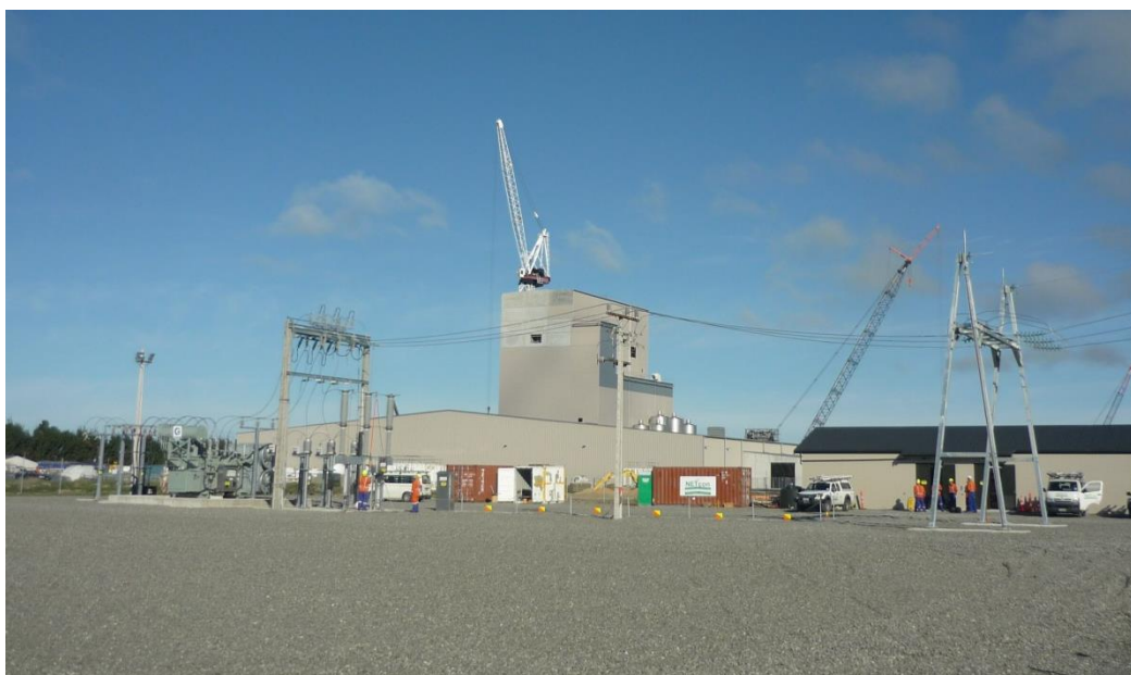
Photograph 3.2 Cooneys Road Zone Substation and Oceania Dairy Limited's Factory
