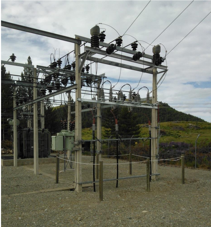
Photograph 7.2 Tekapo Zone Substation
