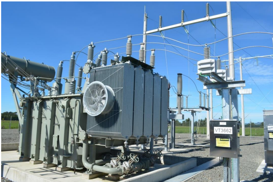
Photograph 3.1 Bell's Pond GXP and Zone Substation
