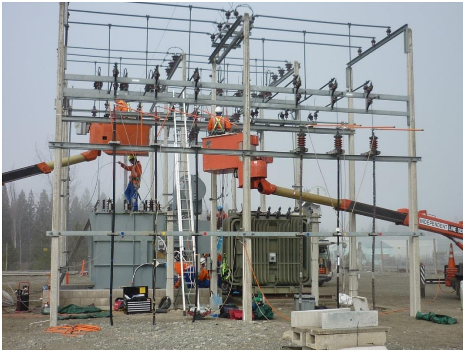
Photograph 10.1 Twizel Village Zone Substation Maintenance—Transformer Swap-out Day
