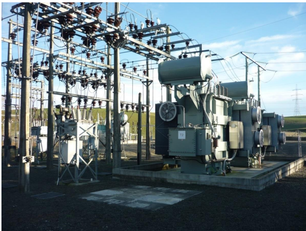
Photograph 9.1 Timaru Zone Substation
