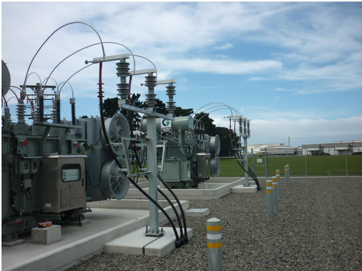
Photograph 9.2 Pareora Zone Substation
