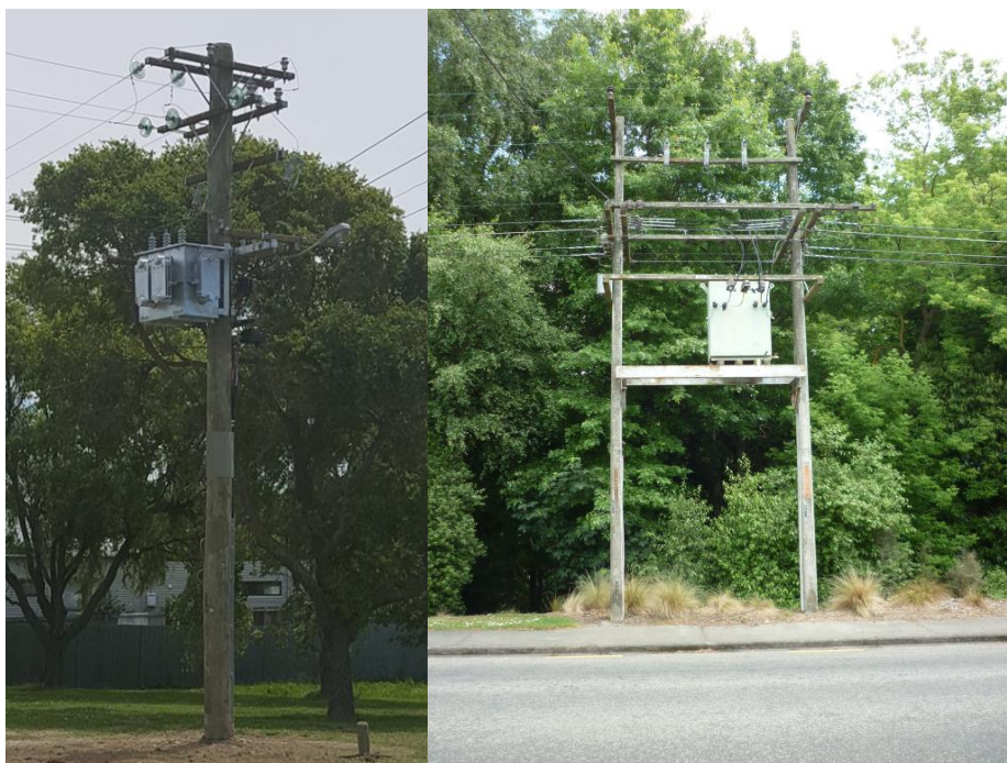
Figure 6-35: Pole mounted distribution transformers
