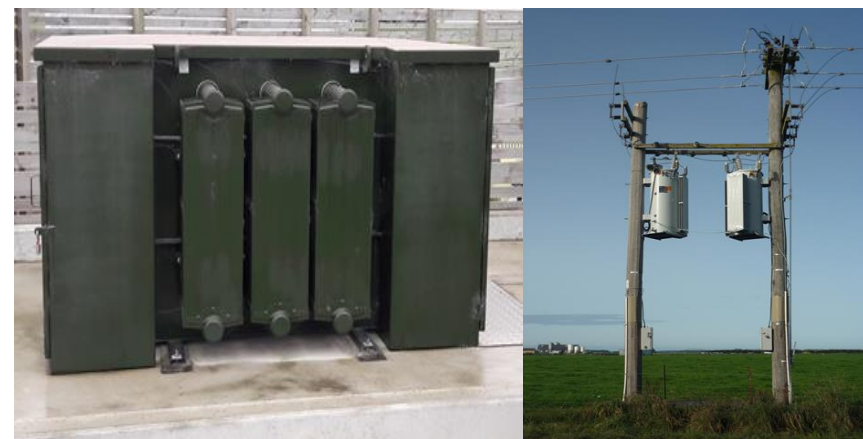
Figure 6-36: Ground mounted transformer (left) and voltage regulator (right)
