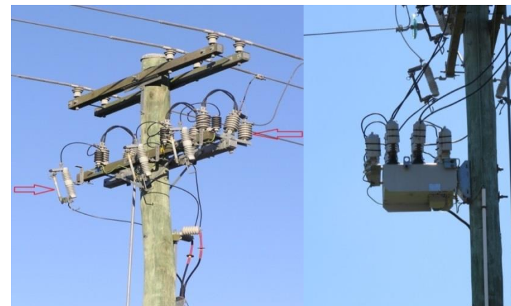
Figure 6-42 Fuse link &amp; ABS left, and a recloser right
