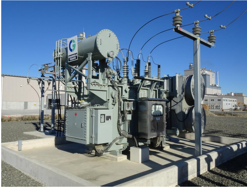
Figure 6-21 Zone substation transformer – Cooneys Road substation
