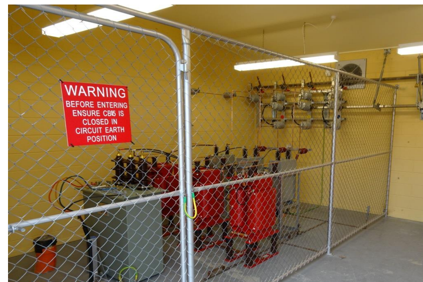
Figure 6-32 Load control injection plant – Bells Pond zone substation
