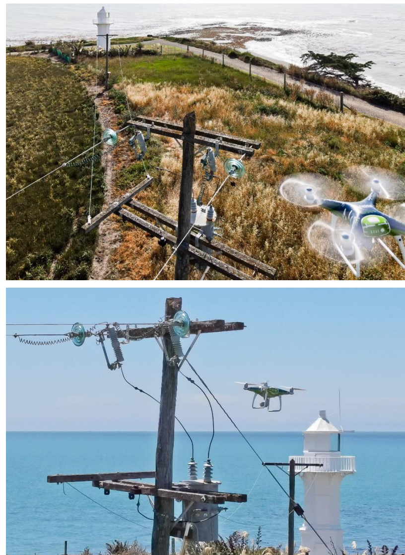
Figure 1-3 Using drones to inspect pole top condition.
