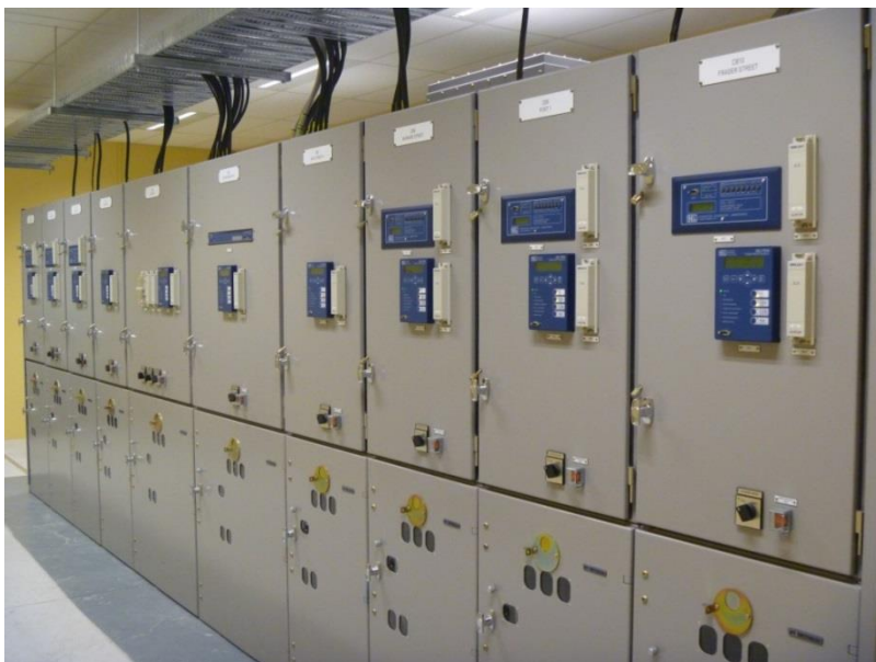
Figure 6-24 11 kV Indoor switchboard at North Street substation
