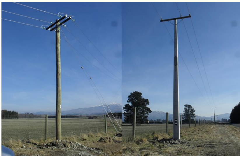
Figure 6-7: Wood pole left and concrete pole right
