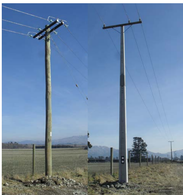
Figure 6.6 Wood pole left and concrete pole right
