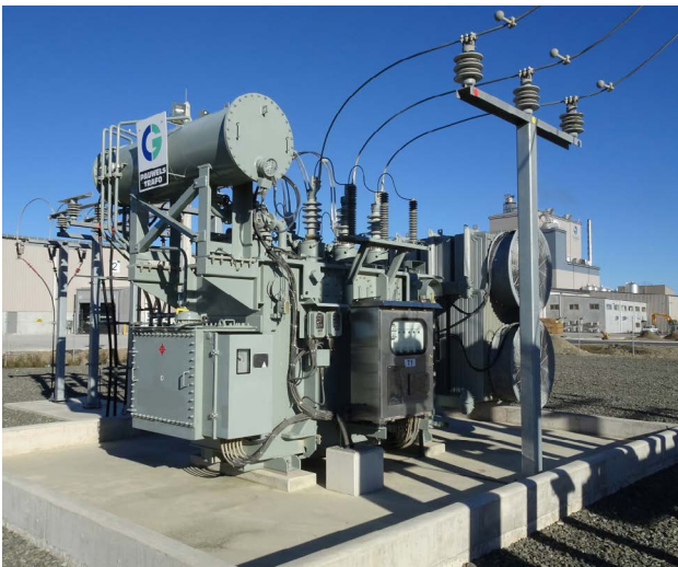
Figure 6.13 Zone substation transformer – Cooneys Road substation
