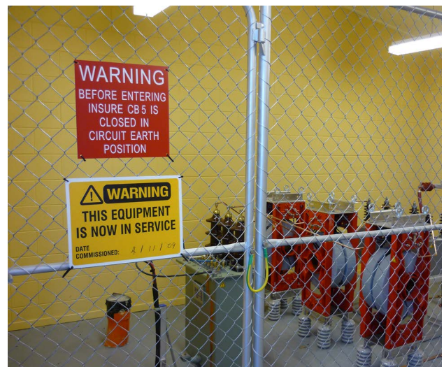
Figure 6.22 Load control injection plant – Bells Pond substation
