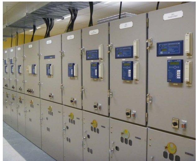
Figure 6.15 11kV Indoor switchboard at North Street substation
