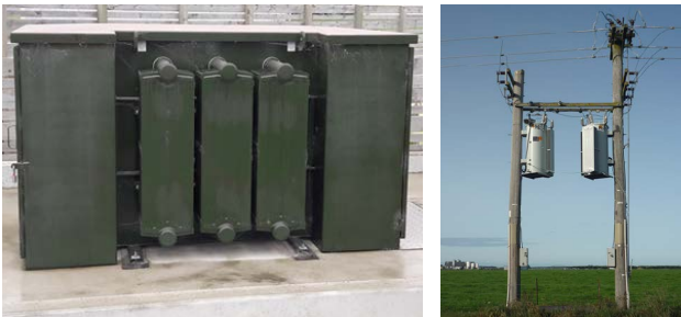
Figure 6.25 Ground mounted transformer (left) and voltage regulator (right)
