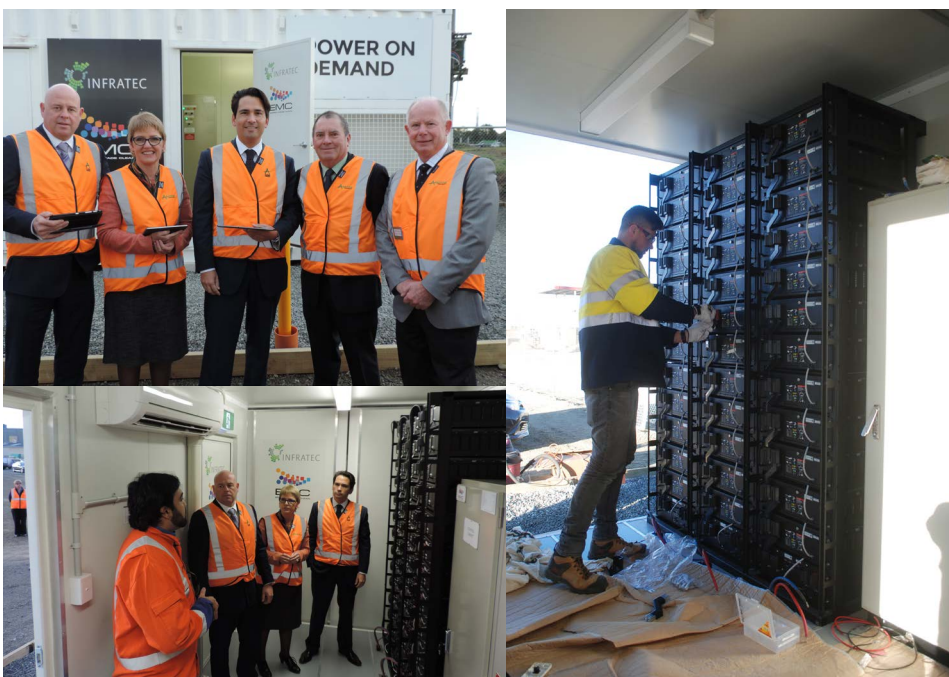
Figure 7.2 Battery energy storage device
