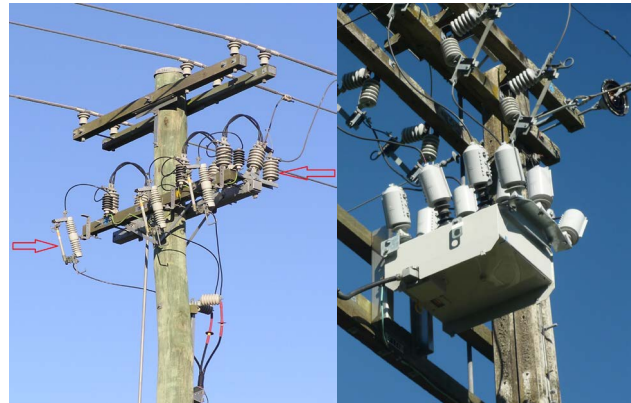
Figure 6.28 Examples of a fuse link and an ABS on the left and a recloser on the right respectively
