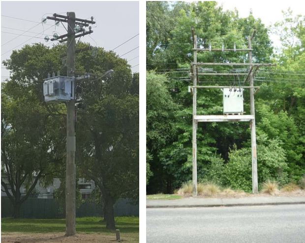
Figure 6.24 Pole mounted distribution transformers
