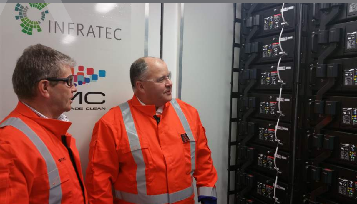
Photo: Infratec/NETcon CEO Steve McCoy and Alpine Energy CEO Andrew Tombs look over the battery storage.
