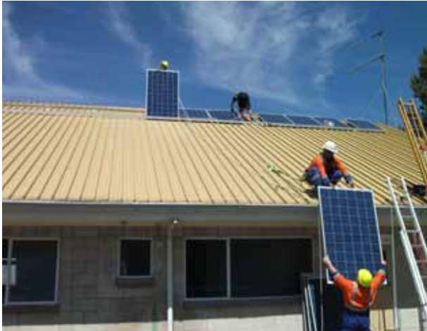
Installing Solar Panels at the Tekapo Substation
