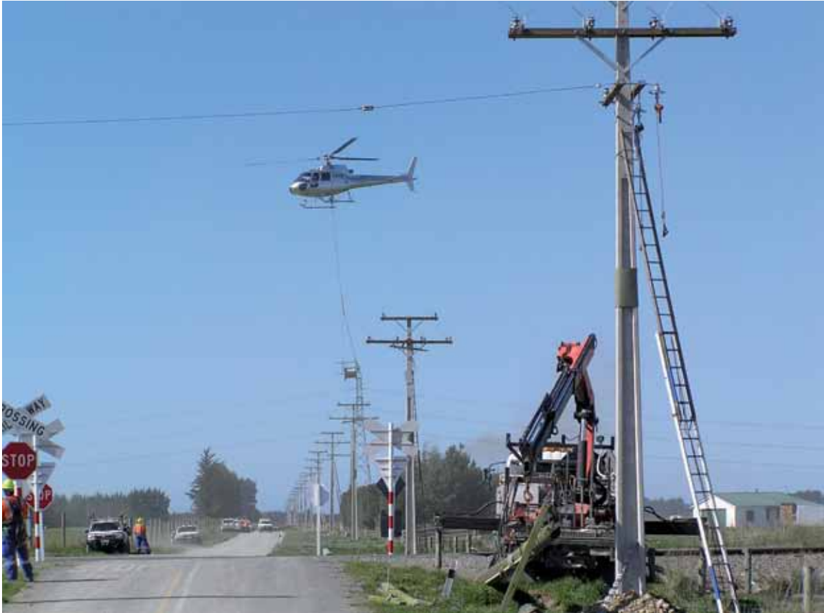
Laying Cables by Helicopter – Rangitata Line
