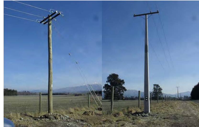
Figure 6-7: Wood pole left and concrete pole right
