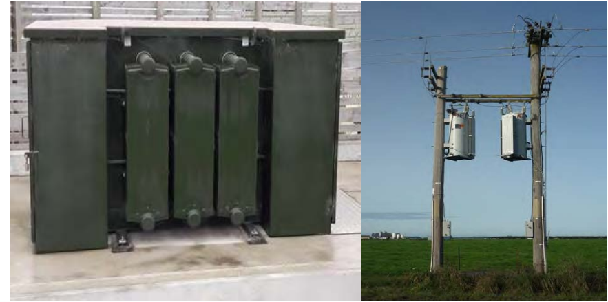
Figure 6-38: Ground mounted transformer (left) and voltage regulator (right)
