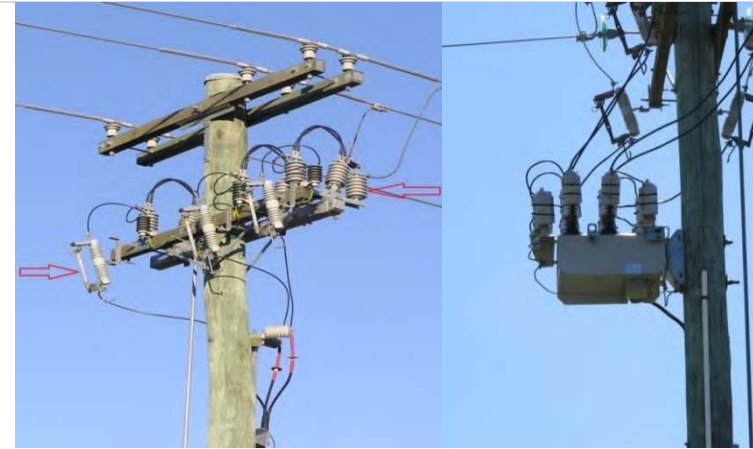
Figure 6-44 Fuse link & ABS left, and a recloser right
