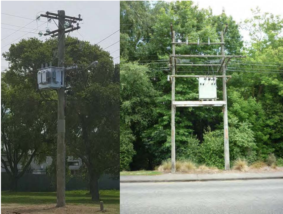
Figure 6-37: Pole mounted distribution transformers
