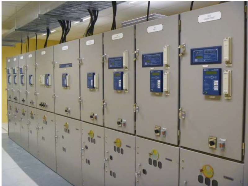
Figure 6-24 11 kV Indoor switchboard at North Street substation
