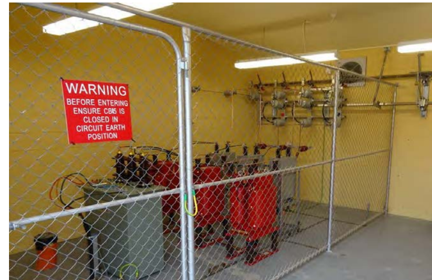
Figure 6-34 Load control injection plant – Bells Pond zone substation
