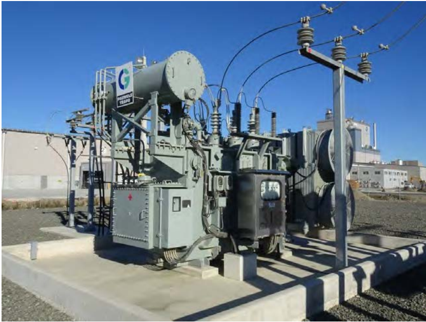
Figure 6-21 Zone substation transformer – Cooneys Road substation
